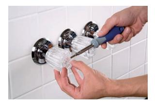
**3.** Use a screwdriver to remove the screw from the center of the handle, and pull off the handle.
