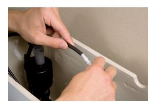
12. Attach the refill tube and adaptor to the overflow valve.
