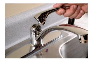
**13.** Reinstall the handle and tighten the setscrew with a hex wrench.
