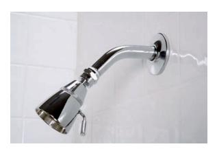
**4.** Cover the showerhead and shower arm with rags to protect them, and finish tightening the showerhead using the adjustable wrench and pliers.
