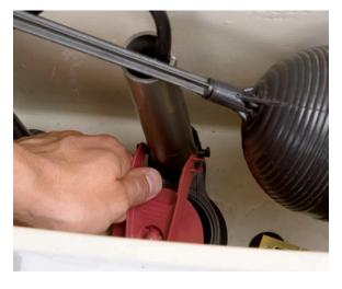
4. Line up the new flapper with the flush valve opening, and slip the flapper tabs over the flush valve ears. The new flapper lift point should be aligned with the flush lift arm.
