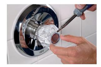
**3.** Use a hex wrench or screwdriver to remove the screw that secures the handle to the cartridge, and remove the handle.
