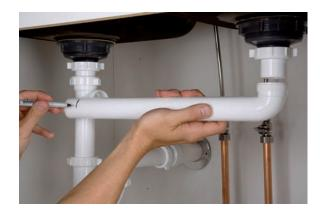
**9.** Slide the slip nut and nylon washer onto the cut end and insert the cut end into the tail piece. Tighten the slip nut.
