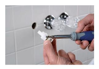
**10.** With a screwdriver, pry the O-ring from the cartridge.
