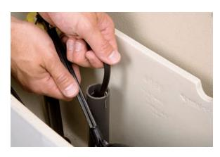
**4.** Disconnect the rubber fill tube from the fill valve that's connected to the flush valve's overflow tube.
