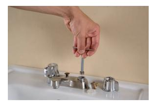
**6.** If the washer seat, which is located inside the faucet handle body where you pulled the stem from, is worn, replace it. Use a seat wrench to unscrew it — don't try to pry it out or you'll damage the faucet body.
