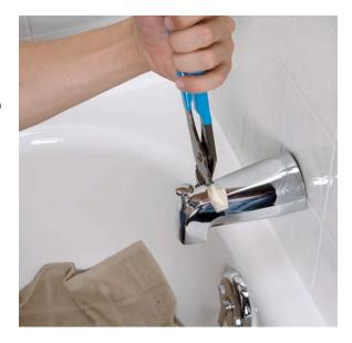
**6.** Finish with a bead of caulk between the spout and tile (see the project "Caulking the Tub, Tile, and Fixtures").
