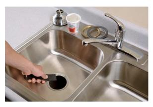
**3.** Scrape off any old plumber's putty on the upper side of the sink with a plastic putty knife. *Don't* use a metal putty knife or you'll damage the sink's finish! If you plan to reuse the old basket, scrape off any old putty under the basket flange.
