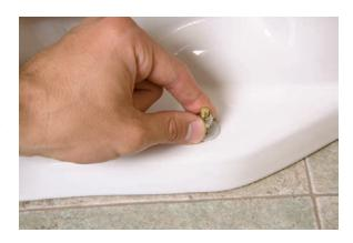
Reinstall the bowl nuts connecting the base to the floor, and tighten them by hand until snug.
