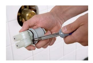
**9.** Rub a thin coat of silicone grease on the new seats (they should be exact replacements of the old ones) before installing them.
