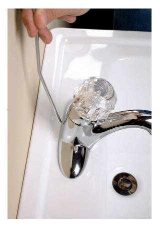
7. Insert the drain plunger lift rod completely through the hole in the top of the faucet. You can adjust the lift height of the rod later.
