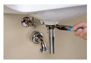
**9.** Use groove-joint pliers to tighten the locknut until it feels snug.
