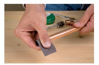
**3.** Use emery cloth to clean the outside of the copper pipe. Clean the pipe to about the width of the emery cloth. Use a reamer brush to clean the inside of the pipe.
