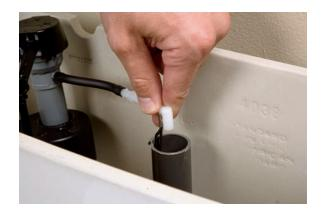
**14.** Remove the valve top cover or cap. Hold an overturned cup over the uncapped valve, and turn on the water supply to flush the system. Flush the system for about 10 to 15 seconds, and then turn off the water. (You want any debris or rust that may have broken loose when you removed and replaced the valve to be flushed out.)
