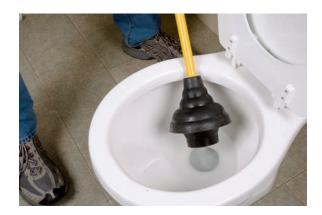
**2.** Place the flange of the plunger over the drain outlet and press down to form the seal.
