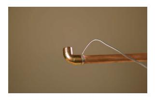
8. Touch the end of the solder wire to the joint created by the pipe and fitting as you continue heating the fitting with the torch. If the solder melts, the pipe is hot enough and ready to solder. If the solder doesn't melt on contact, continue heating the fitting for a few more seconds and then touch the solder to the joint again to check the heat.
