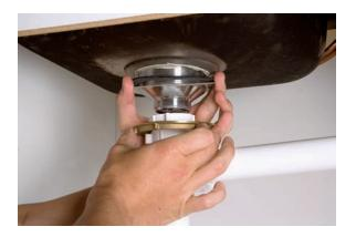
**6.** On the underside of the drain basket, install a new rubber drain gasket and drain seal, and secure them with the locking nut. Handtighten the locking nut.
