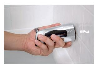
**4.** Screw the new spout onto the threaded supply pipe by hand until it's snug.
