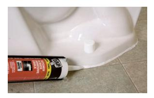
**16.** When you're sure that the toilet is leak-free, apply silicone caulk to fill and seal the gap between the toilet base and the floor.
