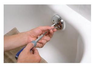
**6.** Tighten the screws on the coverplate. If the drain still won't hold water, repeat the process starting at Step 1.
