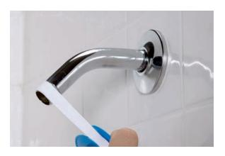
2. Clean the threads of the shower arm with an old toothbrush and then wrap the pipe threads with two or three turns of pipe-thread (Teflon) tape. Wrap the tape in a clockwise direction to keep it from unwrapping when you attach the new showerhead.
