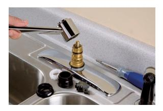
7. Lift the faucet spout straight up off the housing body and set it aside. If needed, clean the faucet body to remove debris. An old toothbrush should do the trick.
