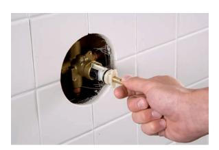
11. Insert the replacement cartridge into the faucet body, making sure it's oriented the same as the one you removed. If your old cartridge isn't in good shape, insert the replacement cartridge.
