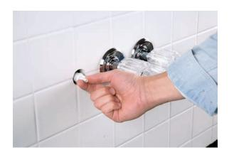
**7.** Remove the cartridge. It should come out by
