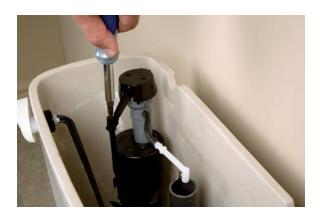
**16.** Adjust the water level in the tank by turning the screw on the rod next to the fill valve. Some fill valves have a clip that you can slide up and down. The water lever should be about 1 inch below the top of the overflow tube.
