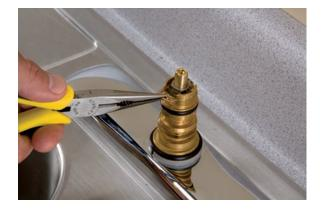
**9.** With the tip of a screwdriver, slip the old Oring from its groove and remove it from the housing. Avoid cutting the ring off the housing so that you can take the old, intact Oring to the store to get an exact replacement.
