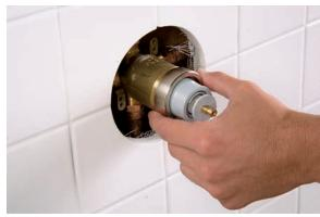
**12.** Place the escutcheon plate over the cylinder and secure it with the three screws.
