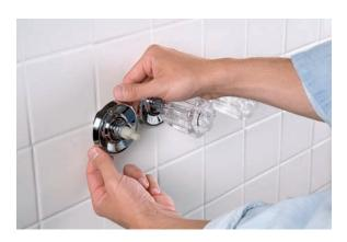
**4.** Remove the escutcheon plate behind the handle body. It should slide right off.
