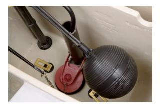
**6.** Adjust the chain length as needed so that there's about ½ inch of slack in the chain.
