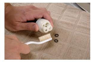
7. Clean the sediment buildup off the seals with an old toothbrush. Also clean out the seal seat area with the toothbrush. If you can't get the sediment and buildup off of the cartridge, replace it.
