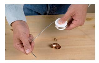
**6.** Unwind the coil of lead-free solder until you have about 8 to 10 inches extending from the spool. About 2 inches from the end, bend the solder at a 90-degree angle.
