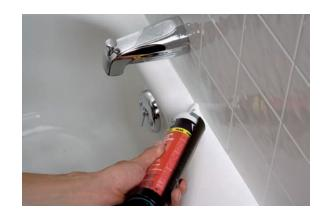
**2.** Apply a bead of caulk around the joint between the tub spout and tile. Rotate the caulk tube in the gun so that you can apply caulk to the underside of the spout joint.
