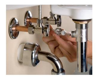
If water leaks from the pivot ball connection: Unscrew the pivot ball retaining nut with groove-joint pliers, and remove the rod, ball, and gasket. Replace the gasket, and reassemble the connection.
