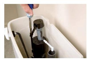
Float cup ballcock: If you have a float cup ballcock valve, lower the water level by turning the screw on the rod connected to the fill valve.
