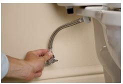
**3.** Disconnect the supply line from the tail piece of the fill valve, located on the underside of the tank. Also disconnect the supply line from the shutoff valve.
