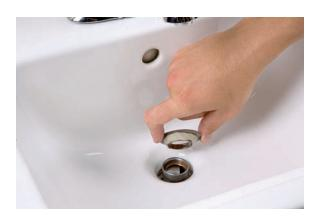
**6.** Thread the flange ring from Step 2 onto the drain body from above. Scrape off any excess plumber's putty using a plastic putty knife.
