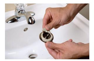
**3.** Screw the drain body and tail piece together. Hand-tighten the locknut onto the drain threads.
