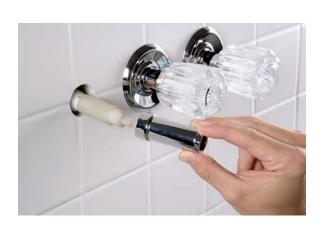
**16.** Slide the metal cover back onto the faucet body and hand-tighten it. Place the escutcheon plate over the metal faucet body.
