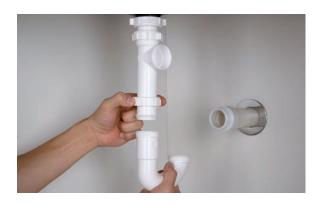
**5.** Position the trap arm on the P-trap, and mark where to cut the arm so that it fits in the wall drain line. Remove the arm and cut it to length using a PVC tube cutter or hacksaw.
