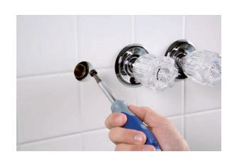
**9.** If the spring doesn't come out when you remove the rubber seat in Step 8, remove the spring with your screwdriver.
