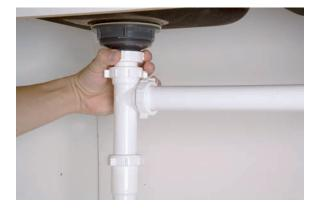
2. Use a basket strainer wrench to loosen and remove the locking nut on the bottom of the basket. (You can try groove-joint pliers first, but most don't open wide enough to go around this type of locking nut.)
