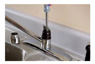
**16.** Reinstall the retaining nut and clip along with the faucet handle.
