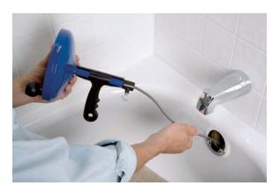
**3.** Push the auger cable into the opening until you feel resistance. Leave about 6 inches of extra cable out of the opening and tighten the auger screw.
