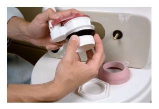
**9.** Install the beveled cone washer onto the tail piece of the new flush valve. The beveled side should face the end of the tail piece. Reinstall the flush valve in the tank.
