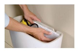
**6.** Press the panel into place against the corresponding side of the tank.
