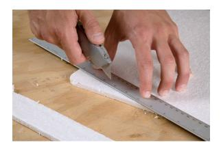
**3.** Cut the foam to the proper width. You may need to angle-cut the bottom corners to fit your tank's contours.
