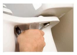
5. Unscrew the tank bolts (one on each side) that connect the tank to the bowl. Use an adjustable wrench to hold the nut located on the bottom of the tank bolt on the underside of the tank (top figure), and loosen the screw with a screwdriver (bottom figure).
