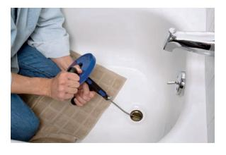
Tighten the auger screw and then turn the auger handle clockwise. Put pressure on the cable as you turn the handle in order to snag or loosen the clog to send it down the drain.
