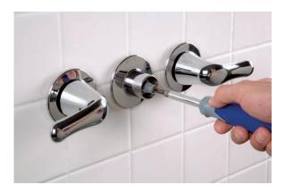
**15.** Tighten the retaining clip.
