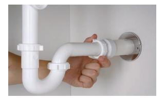
7. Align the arm with the P-trap and tighten; then tighten the arm to the wall drain line.
