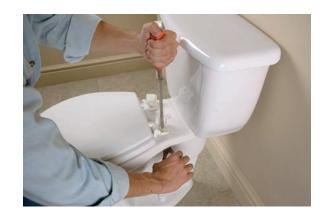
**3.** Align the bolt holes of the new seat with the holes of the toilet base. Push the anchor bolts through the holes, and then screw on the nuts from the underside of the bolts until they're hand-tight.
