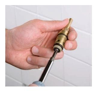
7. If water is dripping from the spout or showerhead, replace the worn washer on the back end of the stem. Remove and save the screw that holds the washer, and replace the O-ring with an exact replacement that you've rubbed with silicone grease.
