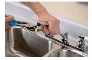
2. Disassemble the aerator by pushing the internal parts out of the aerator housing. A small paper clip might help. If the components are stuck, soak the aerator in white vinegar or lime-dissolver solution (one part vinegar/lime dissolver to one part water) for about 30 minutes or until the deposits are loosened.
