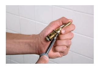
**9.** With your fingertip, rub silicone grease on the new O-ring and insert it on the stem.
