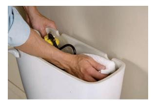
**2.** Hold the foam panel up to the tank and mark how wide the sheet should be to fit within the tank.
