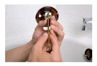
**4.** Screw the rod down about ½ inch and tighten the locknut.
