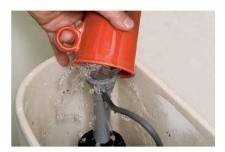
15. Replace the valve cap by engaging the lugs on the cap and valve body and rotating the cap about one-eighth turn. Ensure that the cap is firmly locked to the valve body or you'll have water spraying everywhere when you open the water supply.
