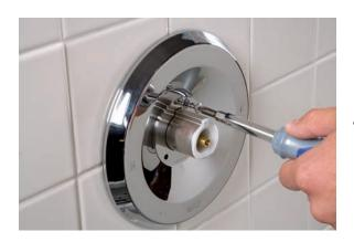
**4.** Remove the screws holding the escutcheon.
