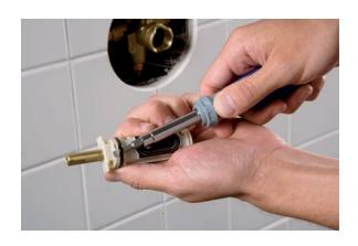
**10.** Rub the new O-rings with a thin coat of silicone grease before putting them on the cartridge.
