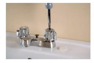
If the handle is stuck, gently tap it with the handle of a screwdriver and try to pry it off again. If it still doesn't budge, use a handle puller to avoid cracking or breaking the handle. (Handle pullers are sold at hardware stores and home centers.)
