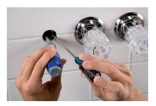
**13.** Use another screwdriver to make sure the parts are pressed in place securely.
