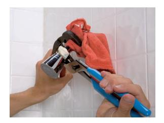
Replacing a showerhead is usually an easy matter of unscrewing the old
